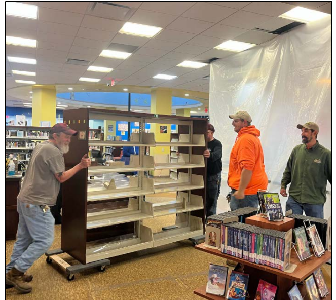
Figure 2 - Public Works helping with renovation
